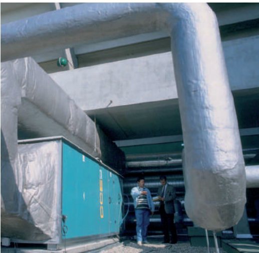
Circulating pumps for building management
