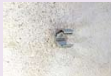
Conduit support is fixed
